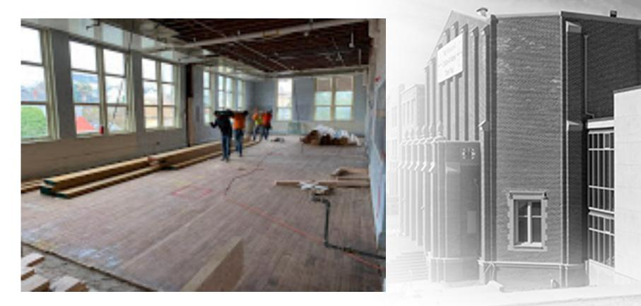
Interior abatement and demolition complete, framing and structural work is underway. New interior classroom walls for reconfigured teaching spaces.
